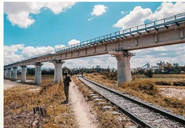
Rail Over Rail Crossing
