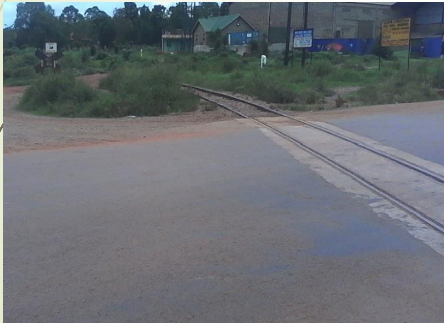
Mukono-Katosi Road Railway level
